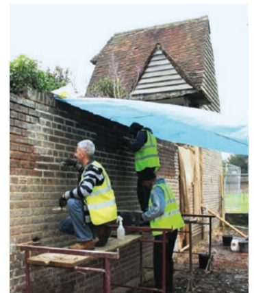
Repair and conservation work in progress
