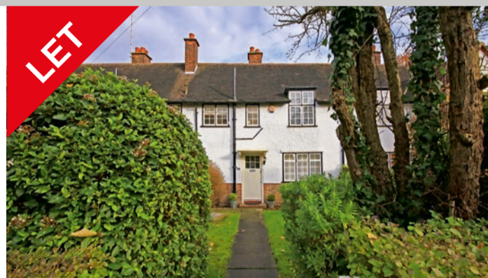
Cottage - Denman Drive North NW11
