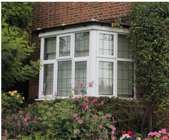
UPVC windows like these detract from the appearance of your house. They are often marketed as being maintenance free. These claims are incorrect. They do not have a long life, they cannot be repaired when damaged and they seriously devalue your house.
