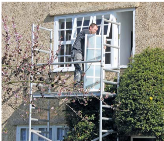
Repairing your existing windows is often the most cost effective option. Adding draught stripping will have a dramatic effect on heat loss and costs very little.
