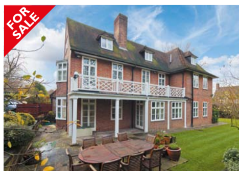
REYNOLDS CLOSE HAMPSTEAD GARDEN SUBURB NW11 Asking Price £2.975M
