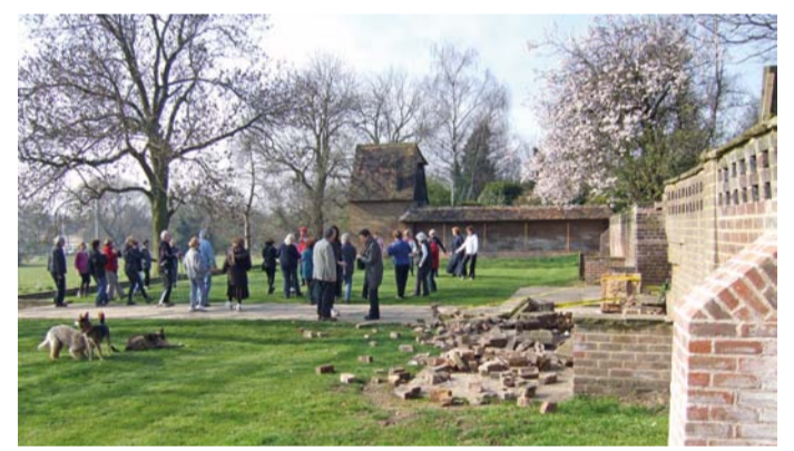
A driver demolished the dwarf wall at the end of Heathgate, along the grass verge adjacent to the york stone path and then crashed into the decorative retaining wall fronting on to the Heath Extension. The car crashed into a section which had been rebuilt in the 1980's and one of the original piers. The pier fell off, but is still partially intact. Sunshine Corner is part of the Grade II listed Great Wall designed by Charles Padget Wade and is the most high-profile public space owned and maintained by the Trust on the Suburb. It has been the subject of a three-year phased programme of repair and conservation by the Trust. The final phase of landscaping to the outer court and areas either side of the york stone path which is due to be undertaken in the 2011/12 financial year, has been slightly delayed by the incident.
