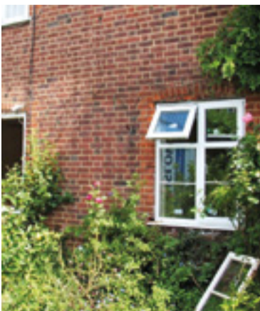
Ripping out timber windows for replacement with upvc is not only illegal but will in fact reduce the value of the property. Such replacements are completely out of character.
