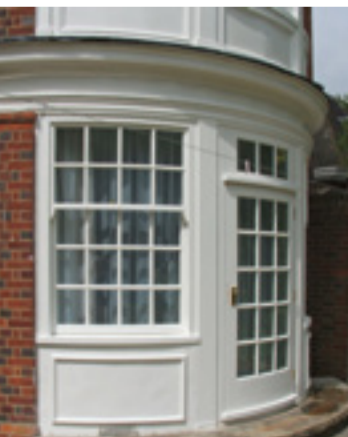
Replacement timber or steel windows can normally be double glazed to enhance the thermal efficiency of your property.
