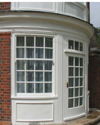
Replacement timber or steel windows can normally be double glazed to enhance the thermal efficiency of your property.
