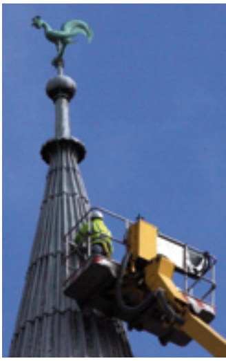
Dramatic repairs. Replacing a five ft. lead panel blown off St Jude's spire.
