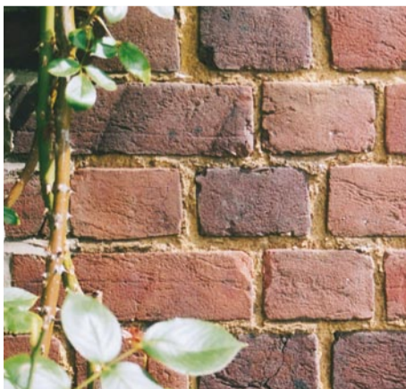
(Unpointed wall) Soft lime mortar weathers naturally, doesn't damage the bricks and has an open texture that allows them to dry out after the rain.
