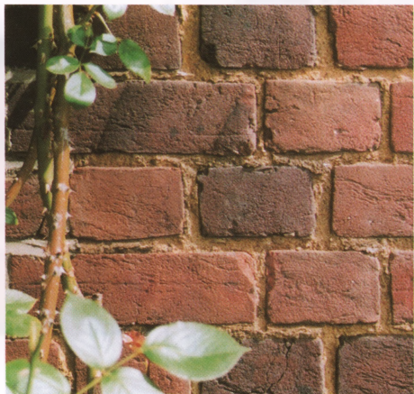
(Unpointed wall) Soft lime mortar weathers naturally, doesn't damage the bricks and has an open texture that allows them to dry out after rain.
