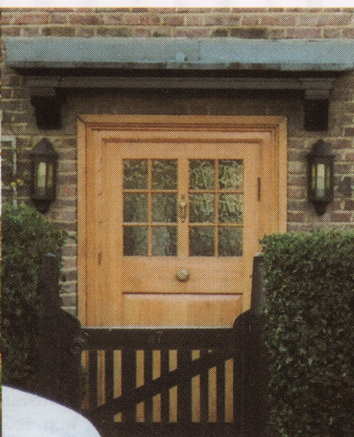
A 'Suburb' door replaced one which spoiled the look of this Hampstead Way house
