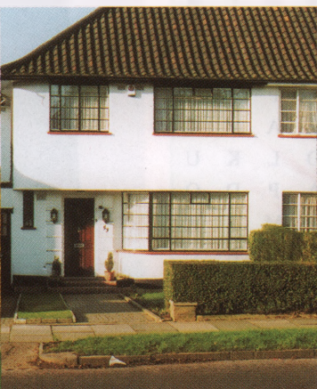
An expanse of paved garden is broken up by the reinstatement of grass and flower beds in Ossulton Way
