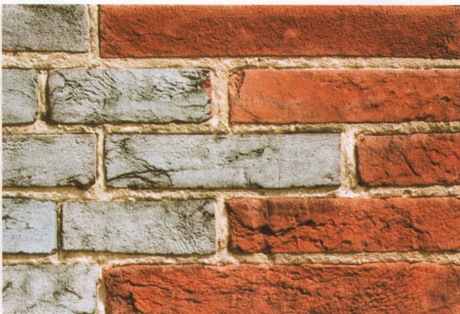
(Unpointed wall) Soft mortar encourages drying out, enhances the beauty of the bricks and makes them less liable to damage when a wet wall freezes.
