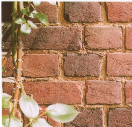
(Unpointed wall) Soft lime mortar weathers naturally, doesn't damage the bricks and has an open texture that allows them to dry out after rain.
