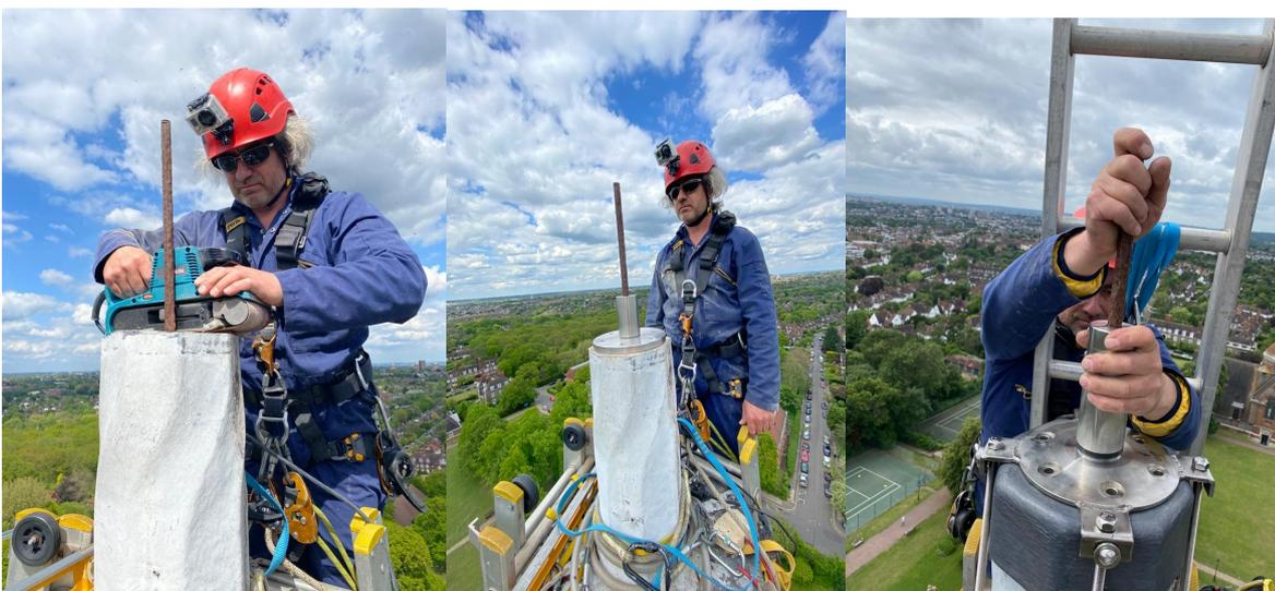
The flanges that have been added to the outer edges of the base serve two purposes, one to help anchor the base to the spire as you can see from the bolts and secondly, to provide connections for the lightning conductor.
