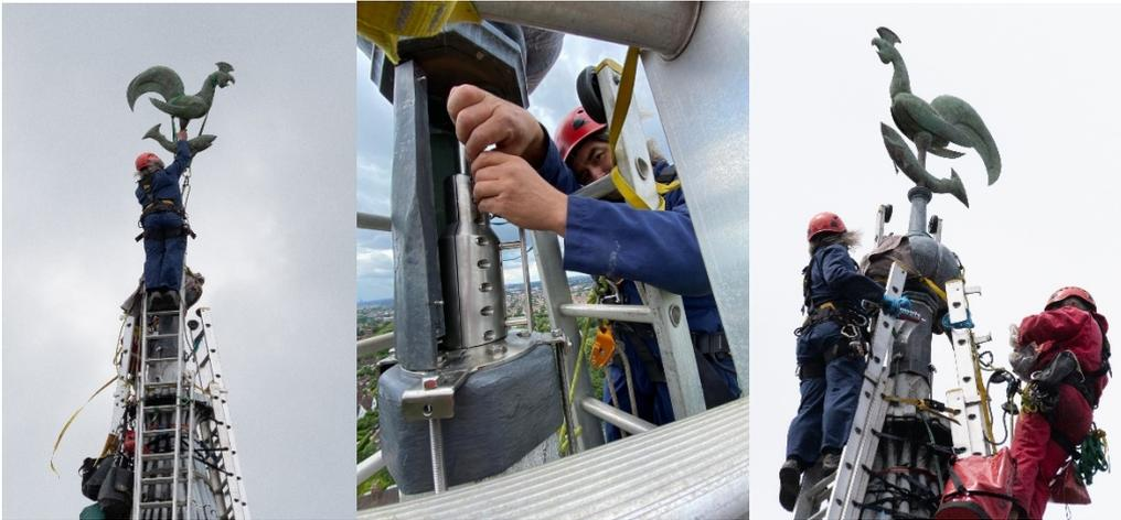
Once the lighting conductors had been reconnected, the ladders that have sat at the top of the spire for the last 4 years were removed.
