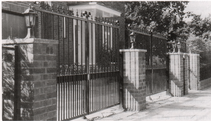
The Trust was about to exercise its legal right to have these gates, which had been put up without planning consent, removed, but before they could do so the house, in Linden Lea, was sold and the new owners agreed to take them down
