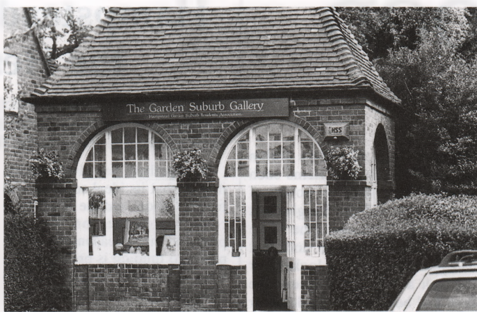
The Garden Suburb Gallery, at the Temple Fortune end of Hampstead Way. The flower baskets are by courtesy of the Temple Fortune Garden Centre
