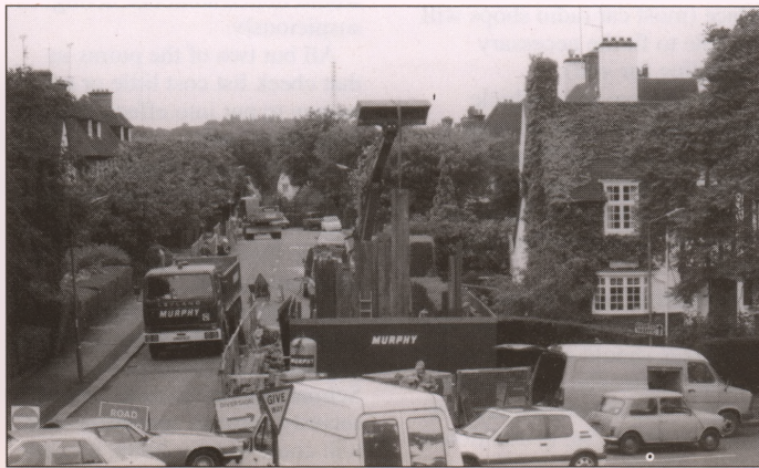
Above: Massive works at the Hampstead Way Meadway Junction where 18' deep shafts are being dug prior to tunneling under Meadway.
