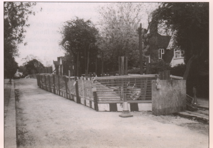
Above: Massive works at the Hampstead Way Meadway Junction where 18' deep shafts are being dug prior to tunneling under Meadway.
