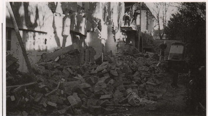
Demolition in progress — men at work.
