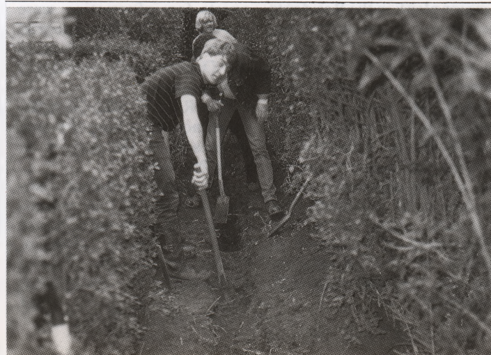
NACRO CP digging up the 'twitten' to the Woodside allotments to enable water to be connected.
