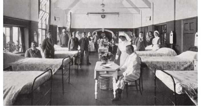
(Above) Ward Garden Suburb Military Hospital Willfield Way
