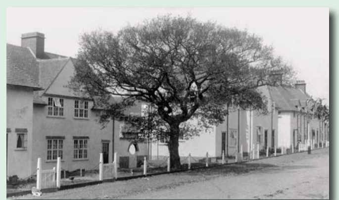
Willifield Way paving
