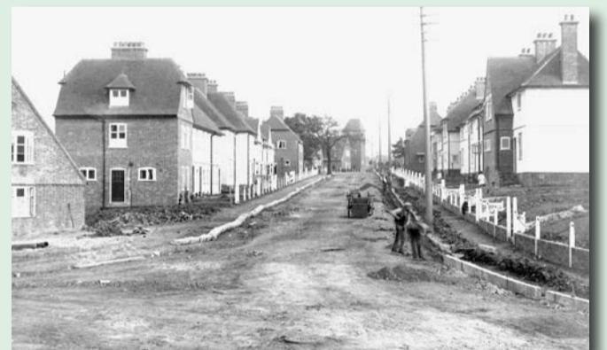
Willifield Way paving under construction
