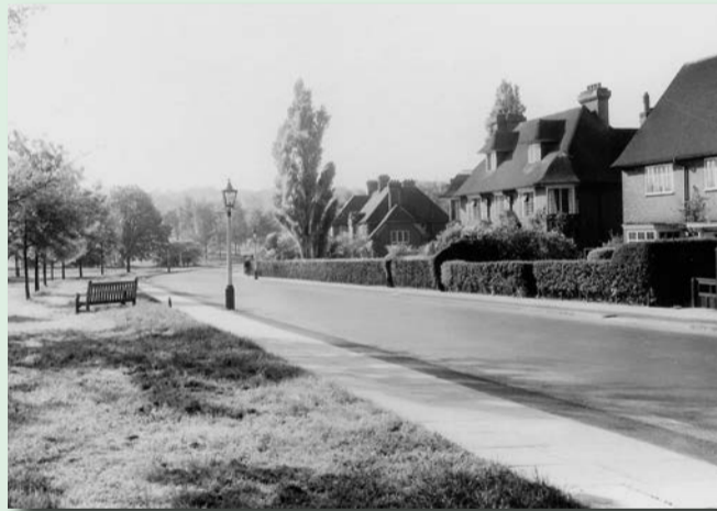
Larger houses on Hampstead Way by the Heath
